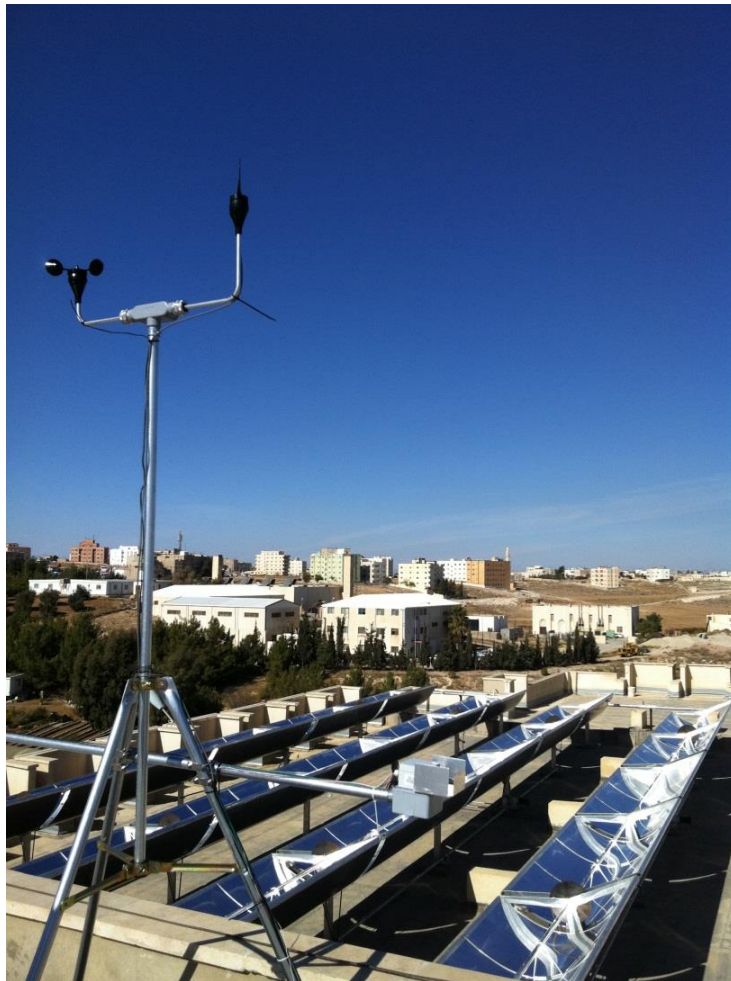
FIGURE 2: MATRIX OF PARABOLIC TROUGH COLLECTORS INSTALLED AT MUTAH UNIVERSITY, JORDAN (SOURCE: MUTAH)
