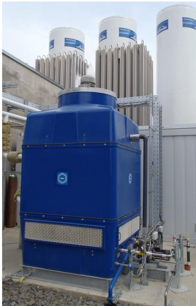
FIGURE 9: EXAMPLE OF WET COOLING TOWER (SOURCE: EWK)
